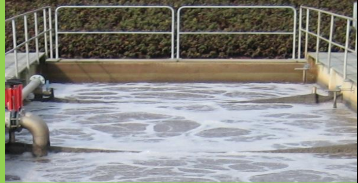
Outlet of the secondary clarifier (exit WWTP)
