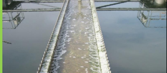
Outlet of the secondary clarifier (exit WWTP)
